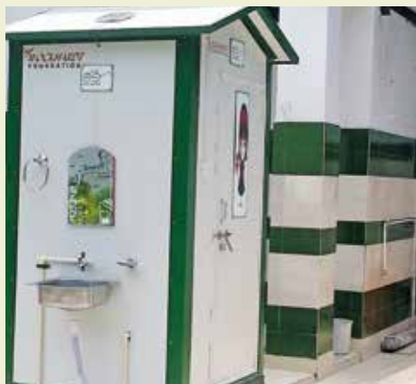
Maurice Nagar, Police Station, Delhi
