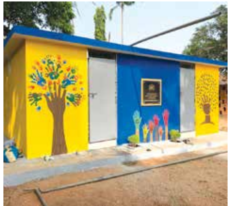
Combined school toilets blocks, Kappu, Udupi District, Karnataka. Partner - BR & CR Shetty Foundation
