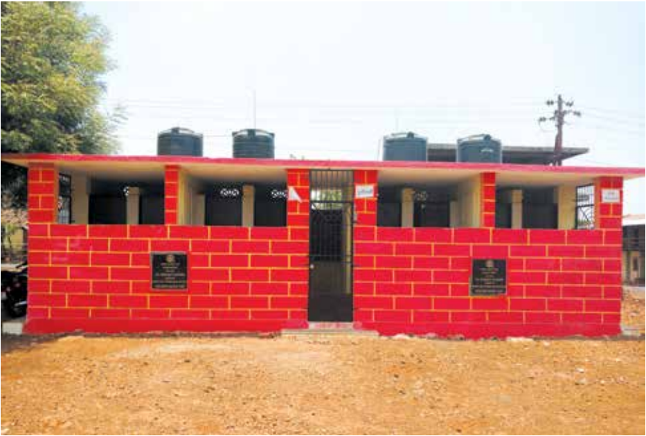
Rotary International, Sukhada Project, Thane, Maharashtra
